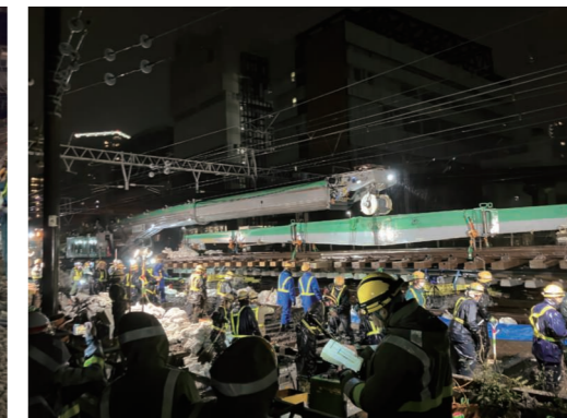
Turnout installation
