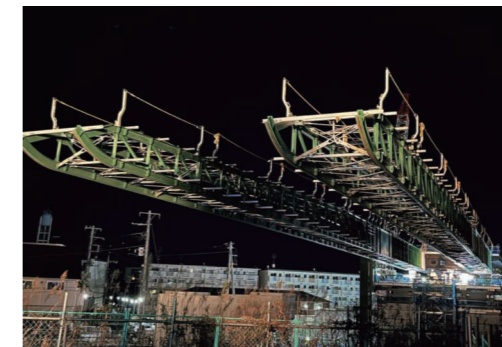
Girder launching with launching nose
