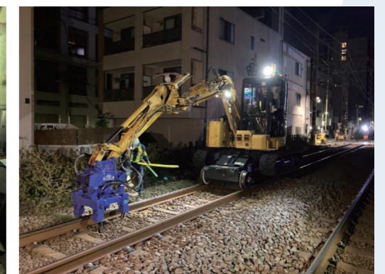
Work with a road-rail backhoe
