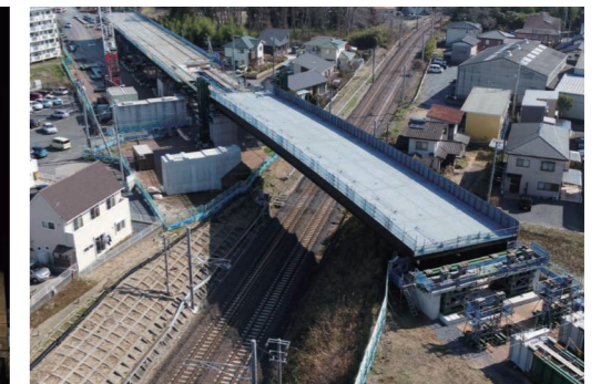
Bridge girder construction was completed by the incremental launching method
